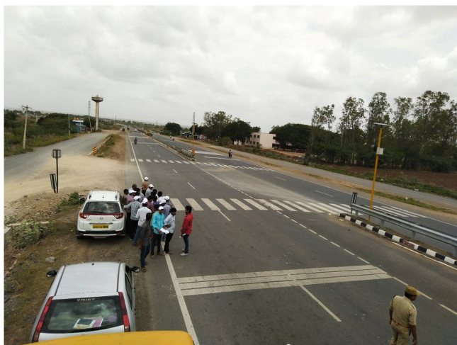
Figure 6.11: Gap In Median
