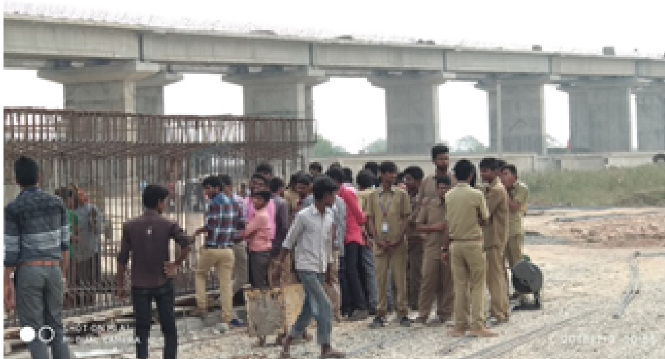
Fig.B.4.5.1.50 Field Visit to Ready Mix Concrete Plant and Bridge Construction at Venkateshwarapuram
